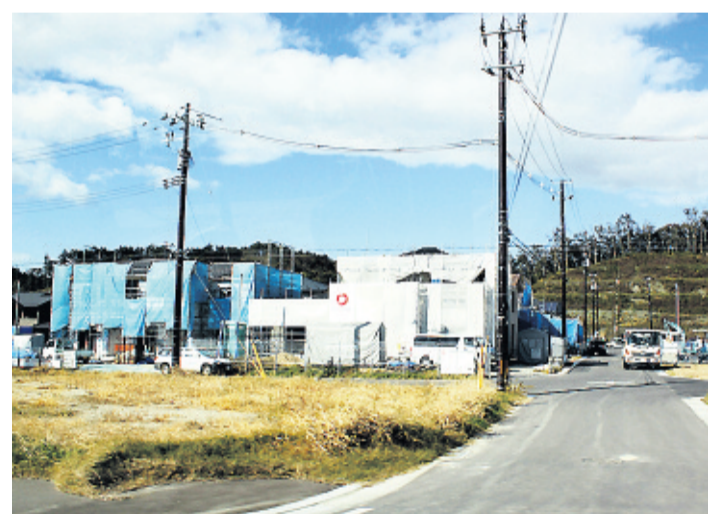
A school under construction in the new city of Higashimatsushima.
